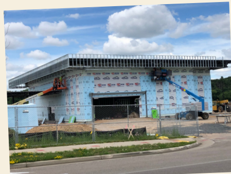
Altoona Office Construction
